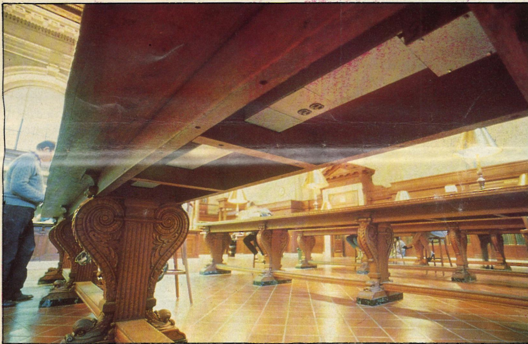
Service runs under reading tables.
